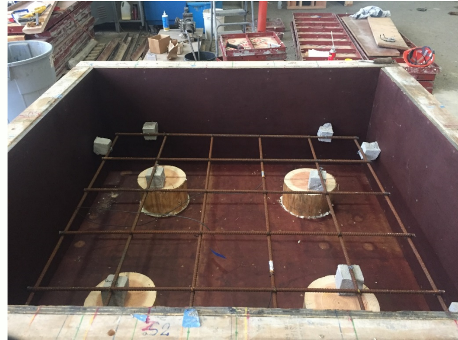
Typical Timber Pile Footing
